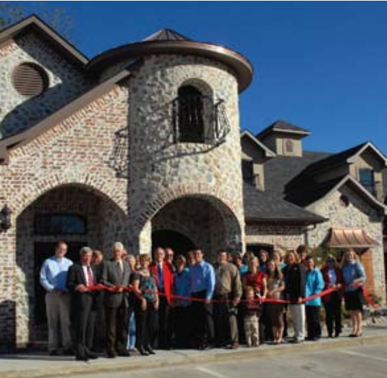
New building for All About Smiles dental offices in Durant, OK. SBA 504 loan provided by REI, Durant, OK.
